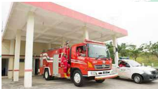
Fasilitas Pemadam Kebakaran Fire Fighter Facility
