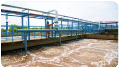
Waste Water Treatment Plant
