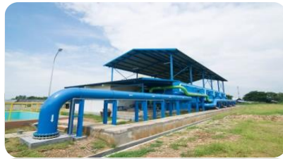
Clean Water Treatment Plant
