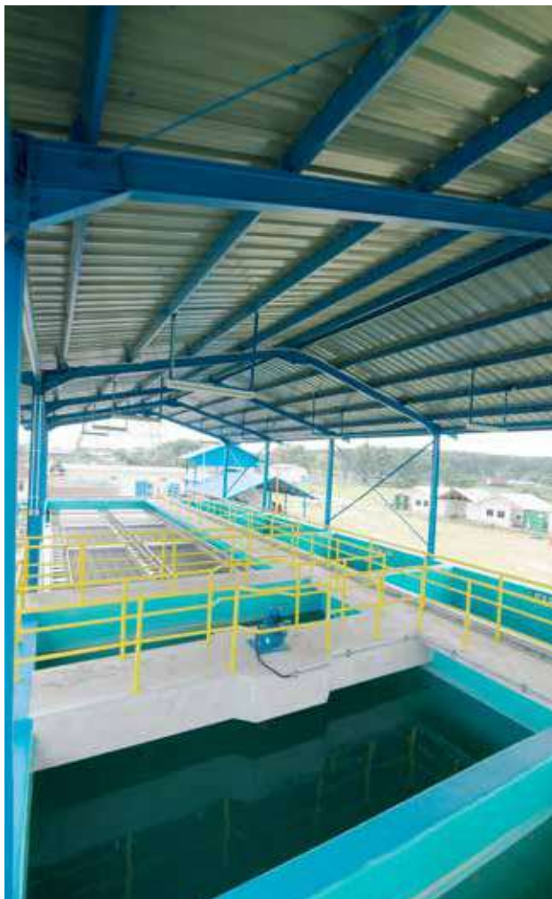
Fasilitas Pengolahan Air Bersih Clean Water Treatment Plant
