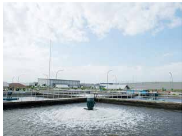
Fasilitas Pengolahan Air Limbah Waste Water Treatment Plant
