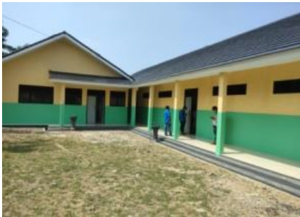
Construction of SDN Cicau 1
