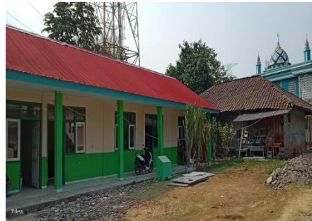
Renovation of PAUD Arumsari
