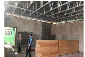
Building Material Donation for the Mosques construction
