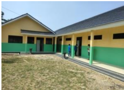
Construction of SDN Cicau 1
