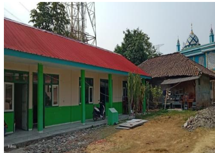
Renovation of PAUD Arumsari
