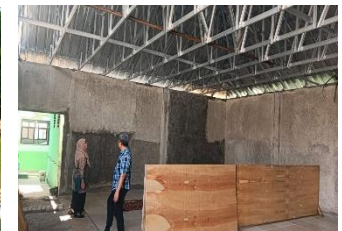
Building Material Donation for the Mosques construction
